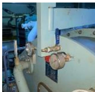
Gambar 2.9 Pressure Vaccum Gauge
