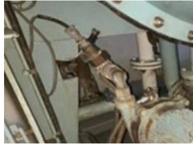
Gambar 2.7 Solenoid Valve
