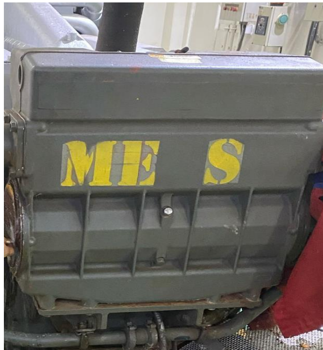
Gambar 2.3: Fresh water cooler
