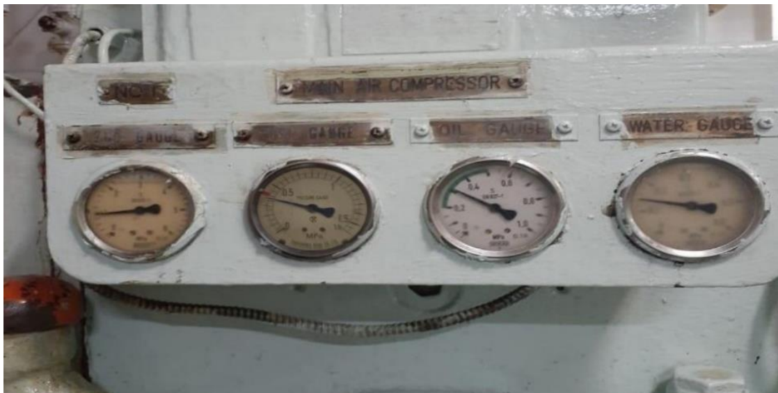
LAMPIRAN 11. Komponen Main Air Compressor TANABE H-64
