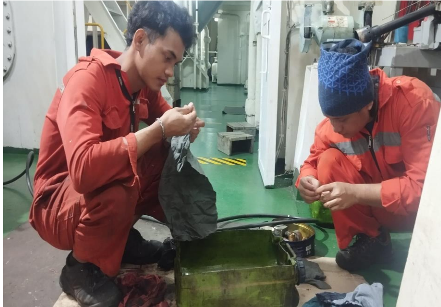
Pembersihan Nozzle Main Burner Boiler
