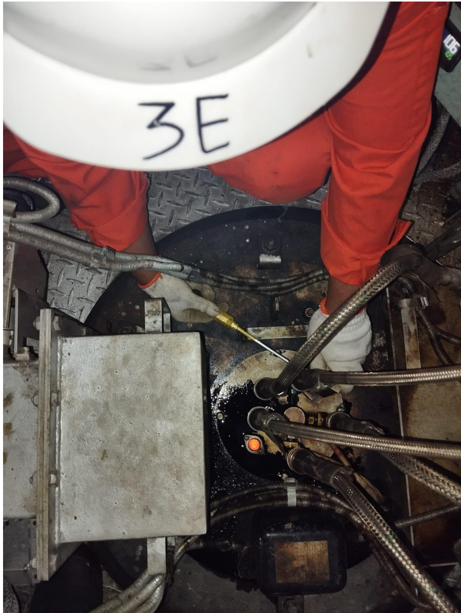
Inspeksi awal Main Burner Boiler
