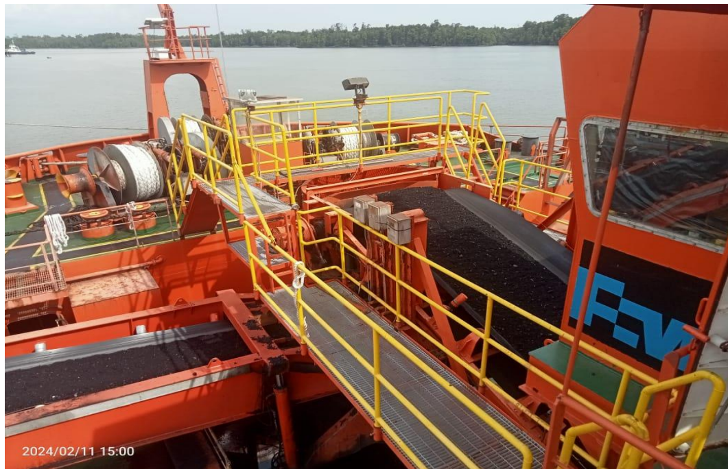
Ship Conveyor system.
