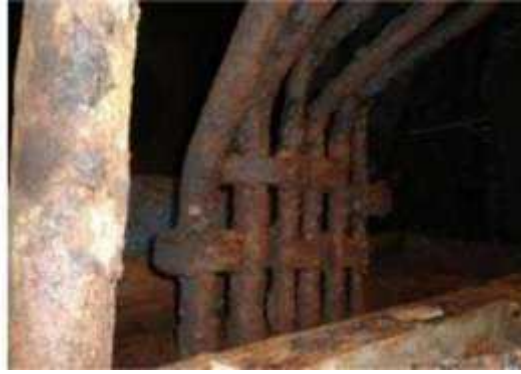
Gambar 2.2 Uniform Attack (Korosi Seragam)
